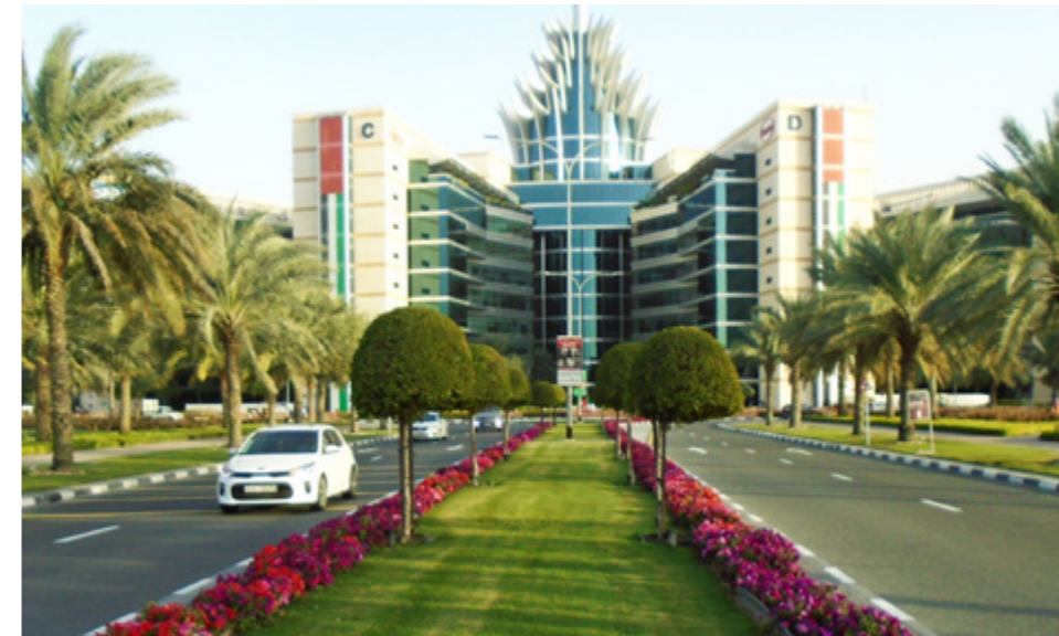
DSO Headquarters, Dubai Silicon Oasis
