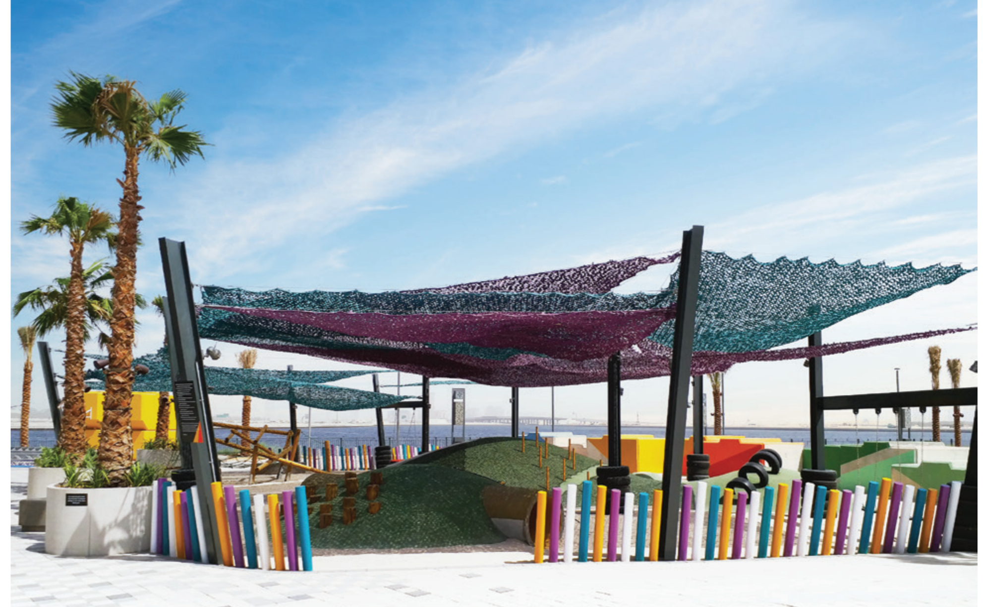
Shade Structure at The Block - Dubai Design District
